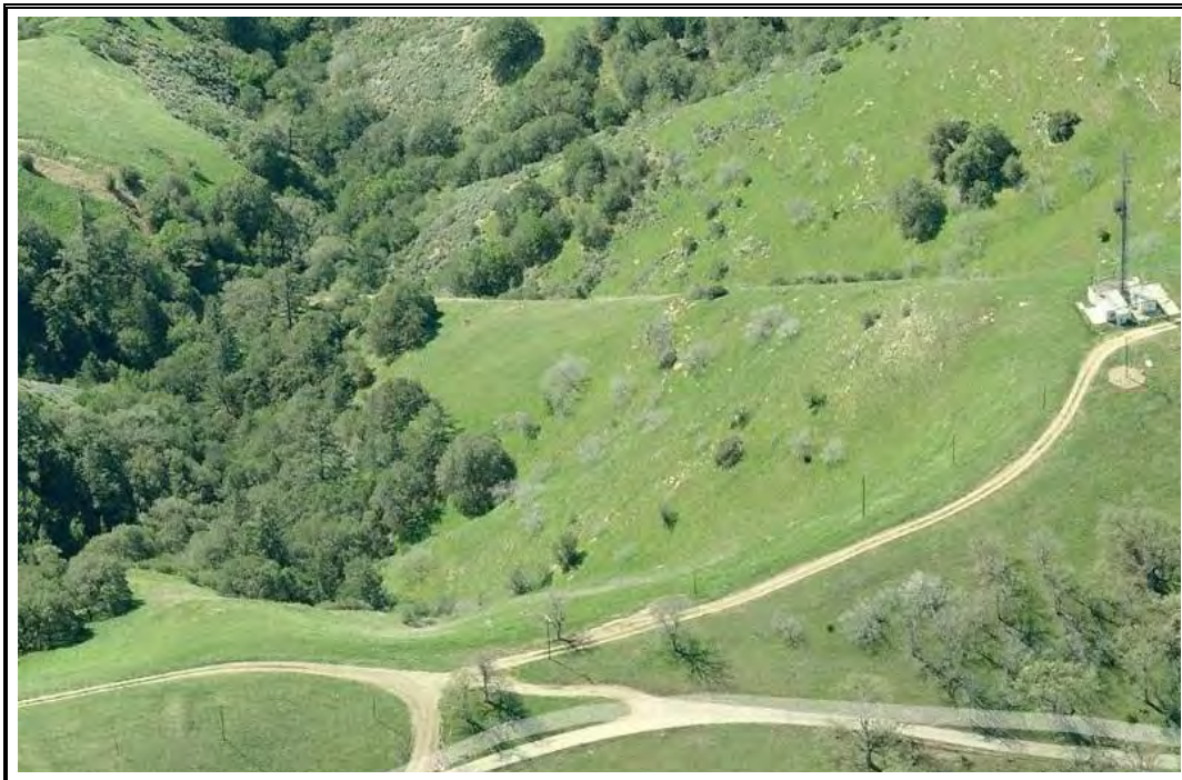
Birdseye view of the west terminus looking south
